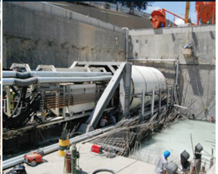
Tunnel Boring Machine
