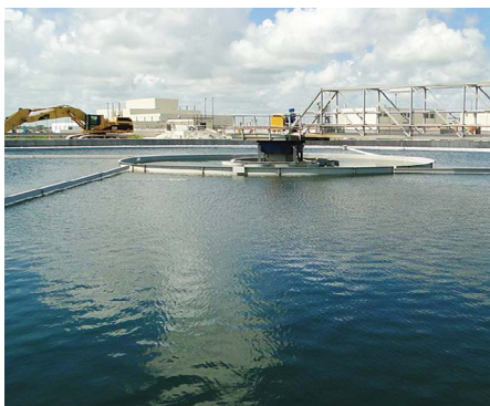
SOUTH DISTRICT WWTP, USA
