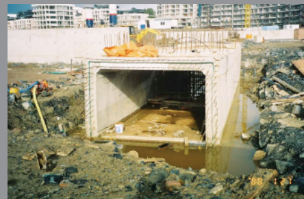
V&A Tunnel, South Africa
