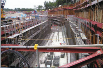
Synchrotron Tunnel, Japan
