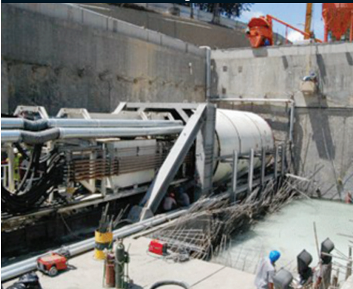
Tunnel Boring Machine
