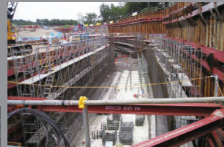
Synchrotron Tunnel, Japan
