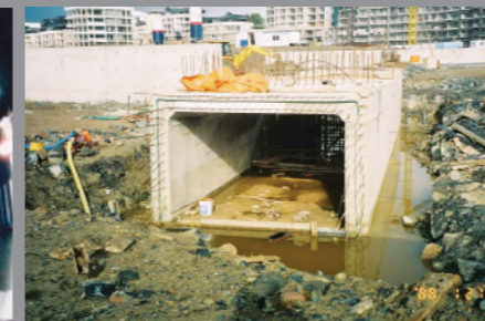
V&A Tunnel, South Africa
