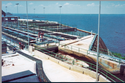
Ponta Do Ismael Water Treatment Plant, Brazil
