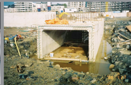
V&A Tunnel, South Africa
