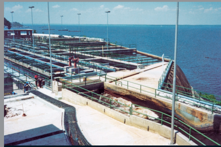
Ponta Do Ismael Water Treatment Plant, Brazil
